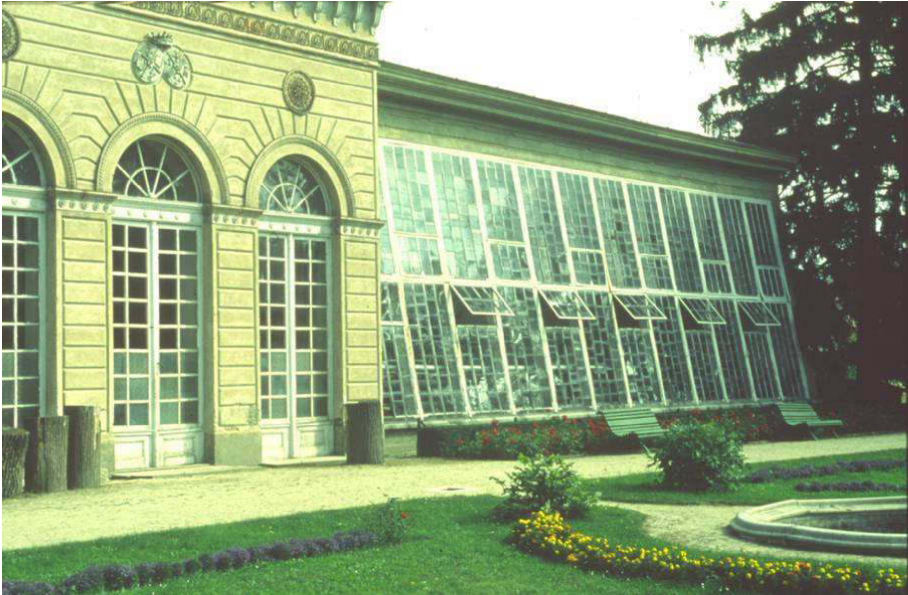
Greenhouse Telc, Czech republic
